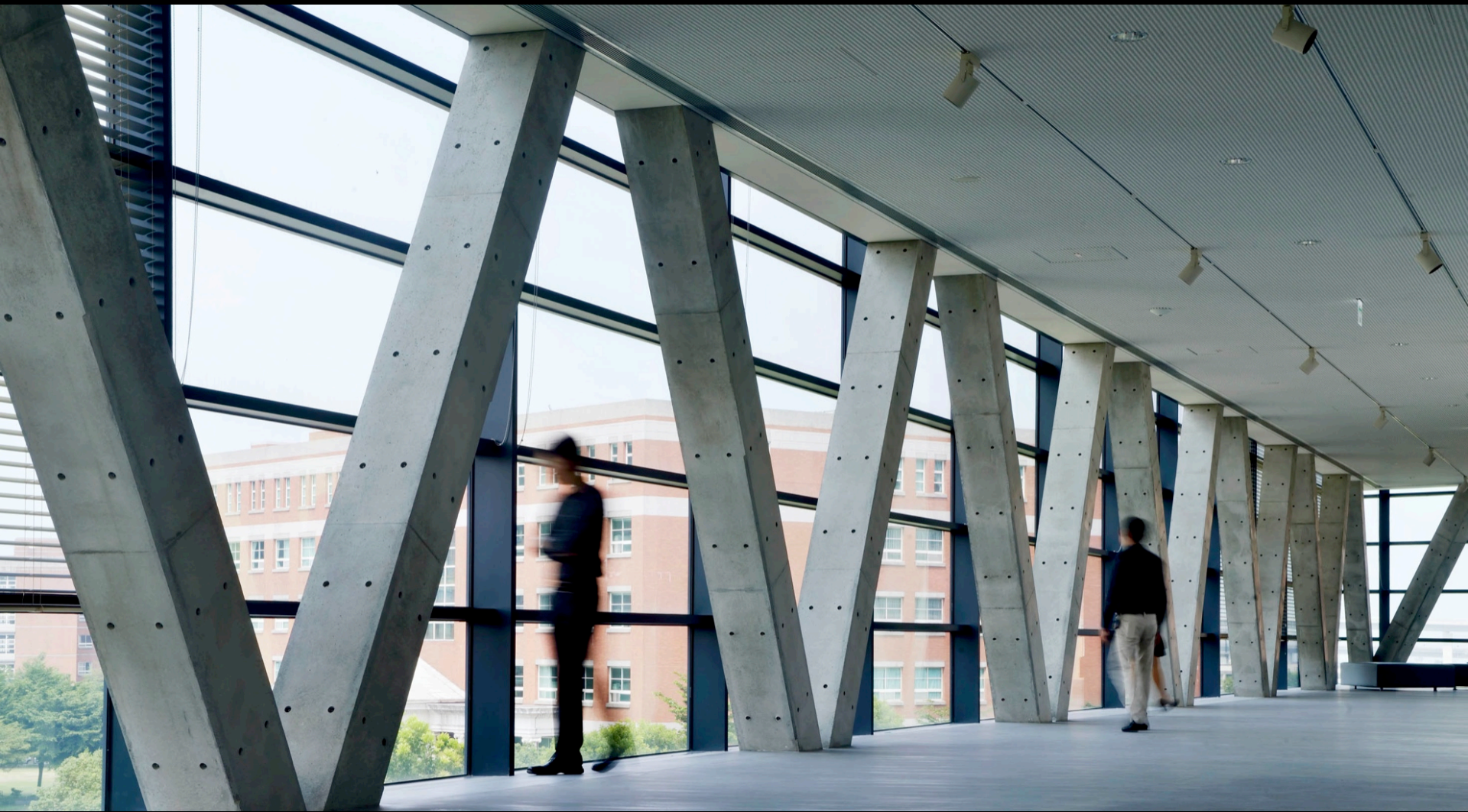
The V-shaped columns and the long-aisle gallery.
